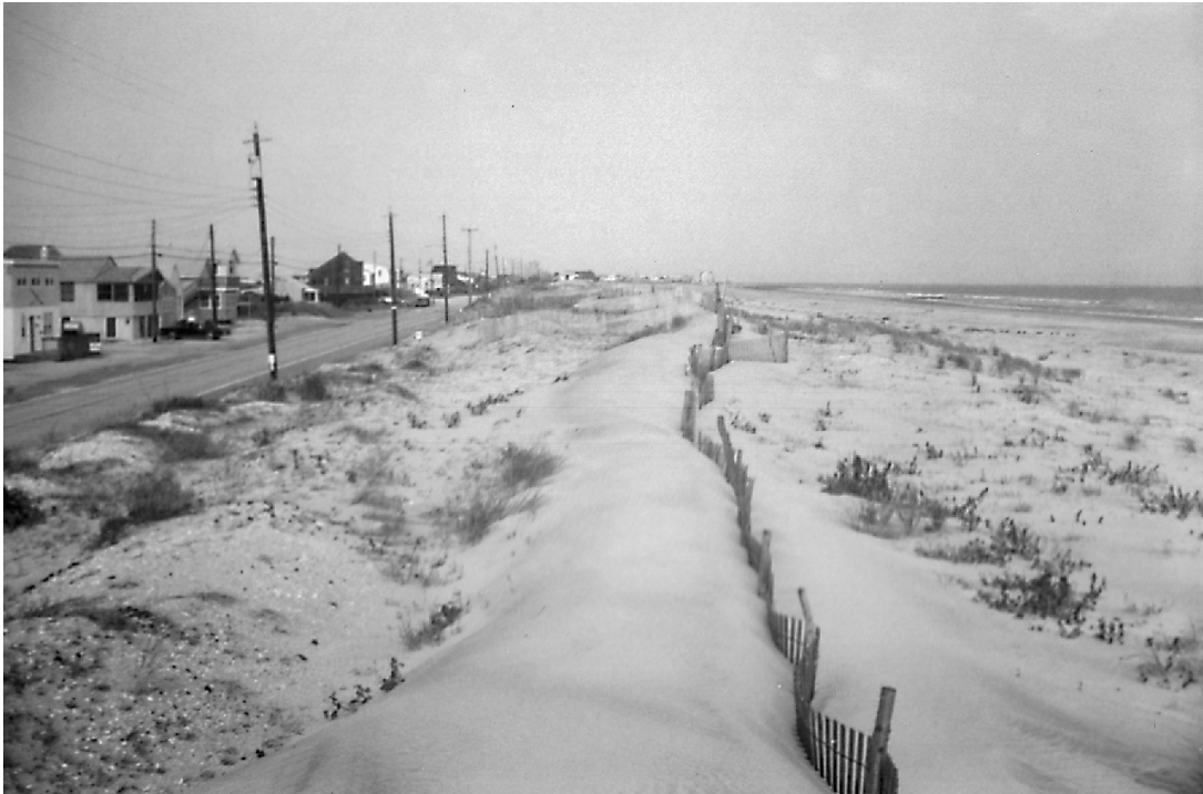
Fig. 4. Artificial dune constructed at Whale beach November 1987 and eliminated in the 1992 storm.
