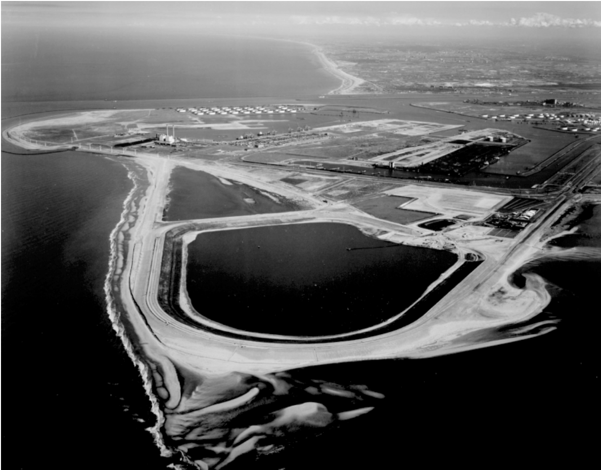
Fig. 6. Building with nature Plan 2 (location see Fig. 1): Land reclamation with industrial uses for the harbour of Rotterdam. In the foreground a depot for polluted harbor sludge. North Sea to the left.
