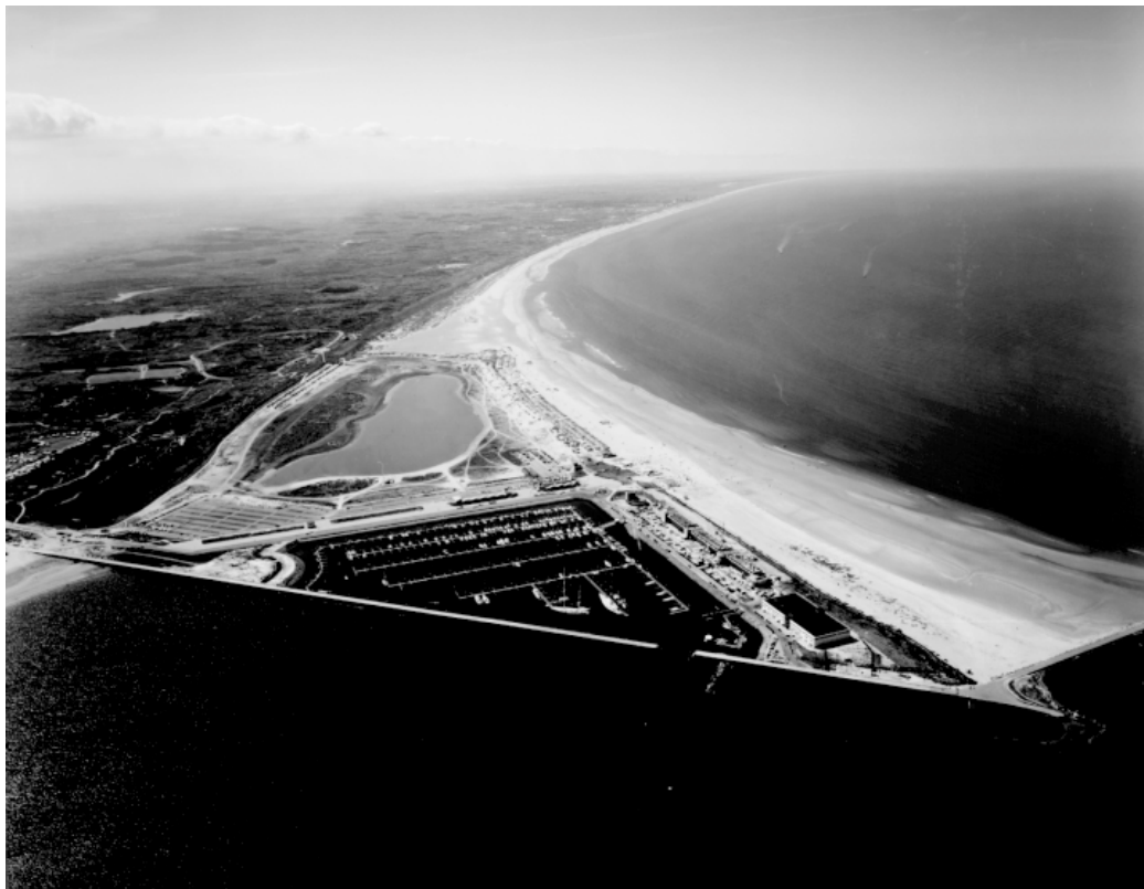
Fig. 8. Building with nature Plan 3: Complete realisation with beaches, initial dunes, lake, marina, car parking and condominiums.
