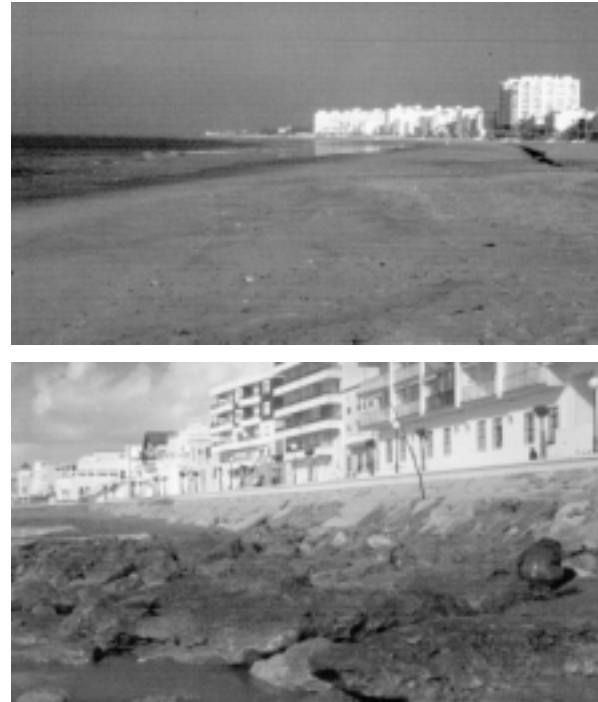
Fig. 4. Rota beach in October 1996, after the nourishment works (a); the same beach after a heavy storm in December 1996, outcropping the rocky substratum (b).
