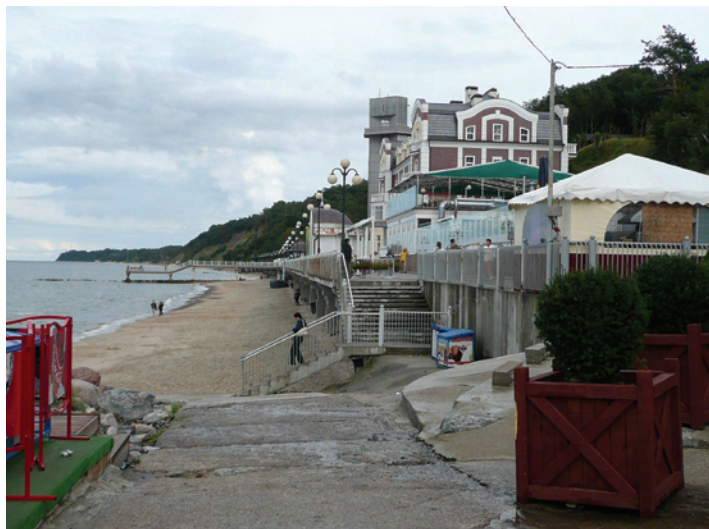
Figure 2: Tourism infrastructure built alongside the eroding cliff coast at Swetlogorsk.
