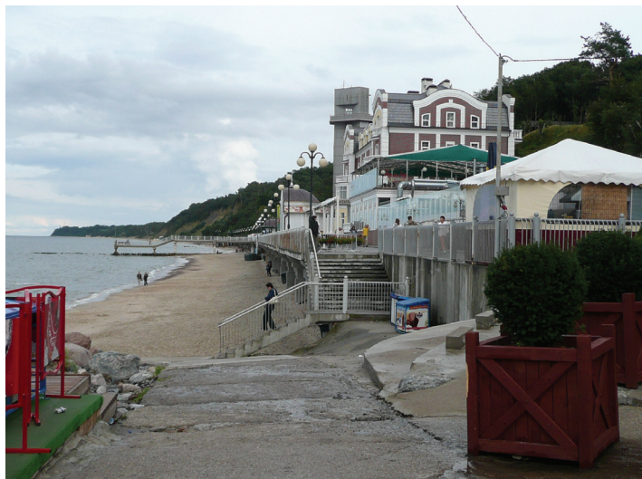
Figure 2: Tourism infrastructure built alongside the eroding cliff coast at Svetlogorsk.
