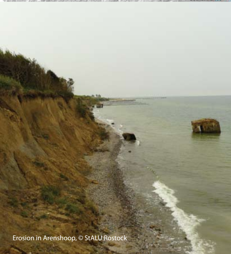
Coastal protection line 2010, © Anja Klee, StALU Rostock
