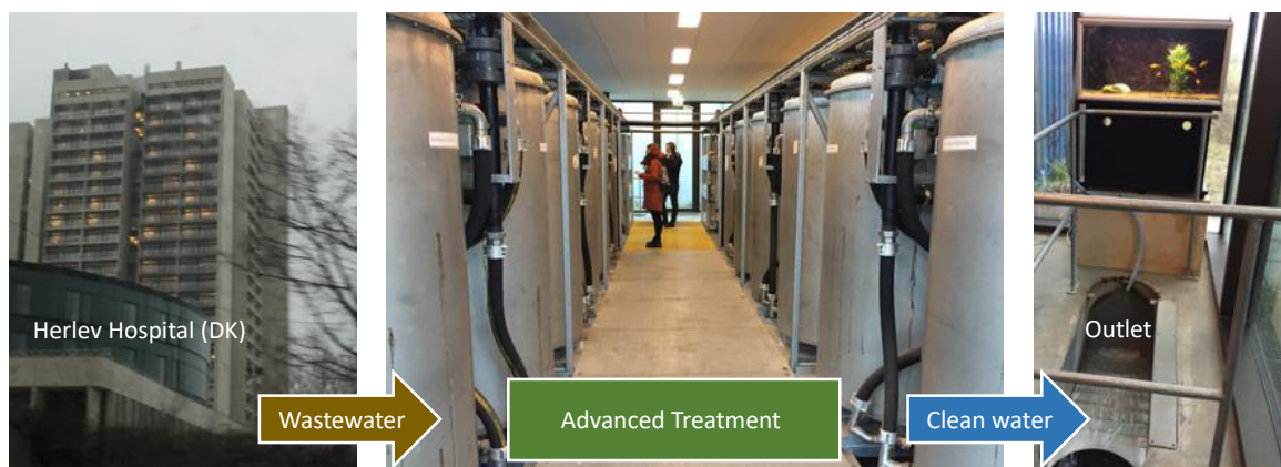
Figure 10. Pictures of the direct treatment of raw waste water from Herlev Hospital Denmark using a combination of advanced treatment technologies reducing the occurrence of pharmaceuticals with more than 99%. Photo: Erland Björklund 2018.
