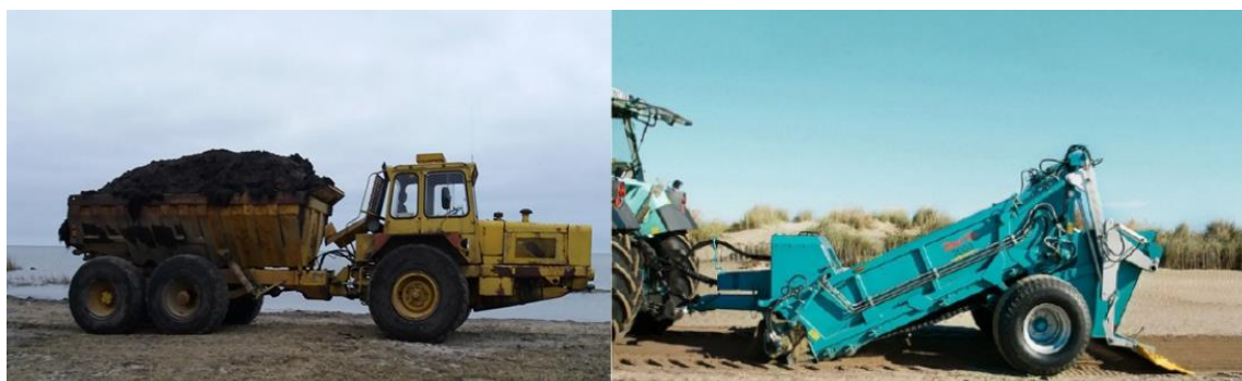
Figure 4.2.1. Beach Wrack removal in Sweden in 2020 (Kalmar) using heavy machinery (W. Hogland).
