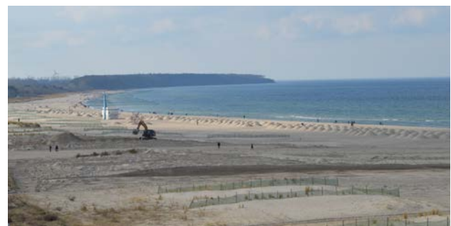
Figure 3.1 Beach management with sand nourishment in Warnemünde, Germany (© EUCC-D) (CONTRA-report Hofmann & Banovec, 2021)
