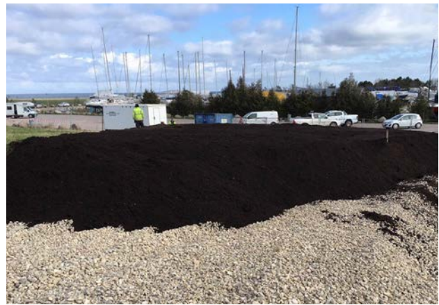
Construction of the biocover at Tangmoseskoven in 2020.
